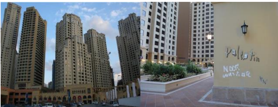
Figure 9. New Gulf project with podium showing vandalism by teenagers in areas obscured from view and car parking
