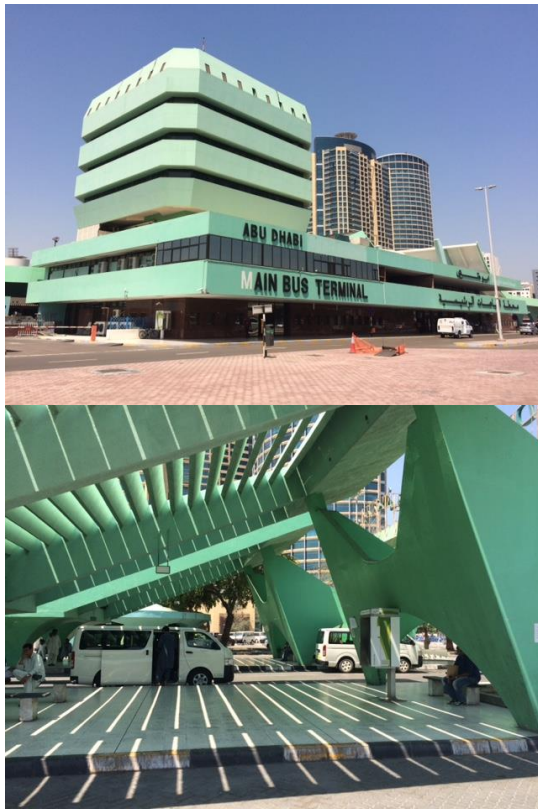
Figure 3. Bus Terminal (top) and Taxi Stand (bottom)
