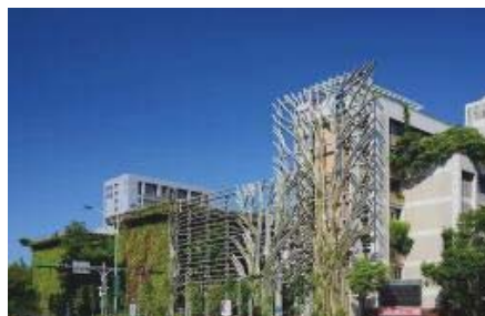
Figure 6. A completed work of the Green Gate
